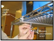
**STEP 13** – USING A FLAT WASHER, LOCK WASHER, AND NUT, SECURE THE SE-4300 EYEWASH UNIT TO THE CENTER CROSS SUPPORT AND TOP SHELF OF THE SAFETY CART.
