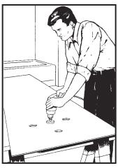
7. Cut holes 1/2" larger than the diameter of the pipes. Drill from the finished side of the panel. For best results place a scrap of wood beneath the hole to be cut, this will give you a clean cut opening.
