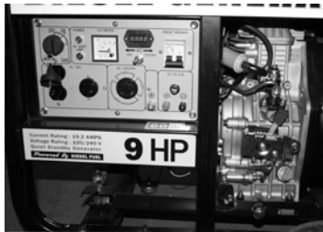
Figure 1 – Front Of Generator
