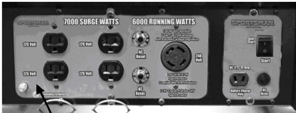
Figure 3 - Attaching the Grounding Wire to this Generator
