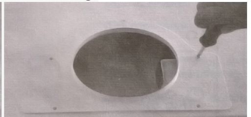
Type 3: 6-inch round vent adapter on top of the range hood.
