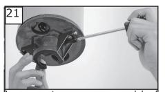
Loosen two preassembled screws across from each other corresponding to the open slotted holes on the canopy upper rim and remove the other two screws from mounting bracket. Keep screws for later use.
