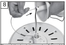
Thread the leadwires and safety cable through the downrod.
