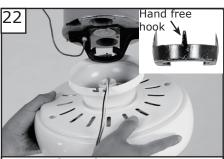
Hang fan from mounting bracket by the hands free hook into a closed hole on the edge of the Canopy.
