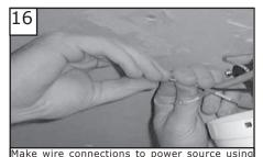
wire connections to power source using wire nuts provided. Make sure that no filiments are outside of the wirenut. After making the wire connections, the wires should be spread apart with the grounded conductor and the equipment-grounding conductor on one side of the outlet box and ungrounded conductor on the other side of the outlet box. The splices after being made should be turned upward and pushed carefully up into the outlet box.
