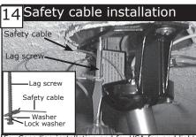
For Canadian installation and for USA fan and light kit combinations over 35 lbs, in both flush and downrod mode the safety cable must be installed into the house structure beams using the 3" lag screws, washers, and lock washers. provided. Make sure that when the safety cable is fully extended the leadwires are longer than the cable and no stress is placed on the leadwires.
