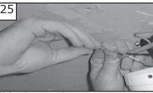
Make wire connections to power source using wire nuts provided. Make sure that no filiments are outside of the wirenut. After making the wire connections, the wires should be spread apart with the grounded conductor and the equipment-grounding conductor on one side of the outlet box and ungrounded conductor on the other side of the outlet box. The splices after being made should be turned upward and pushed carefully up into the outlet box.
