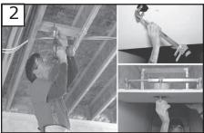
Before installing this fan make sure the outlet box is properly installed to the house structure. To reduce the risk of fire, electric shock, or personal injury, mount to outlet box or supporting system acceptable for fan support.
