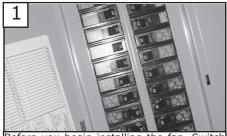
Before you begin installing the fan, Switch power off at Service panel and lock service disconnecting means to prevent power from being switched on accidentally. When the service disconnecting means cannot be locked, securely fasten a prominent warning device, such as a tag, to the service panel.
