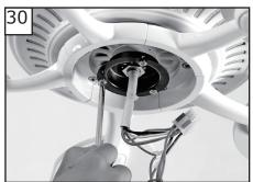
Loosen 2 and remove 1 preassembled scews from the plate on motor. Save screw for later use.
