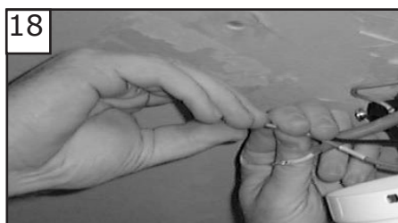
18 Make wire connections to power source using wire nuts provided. Make sure that no filaments are outside of the wirenut. After making the wire connections, the wires should be spread apart with the grounded conductor and the equipment-grounding conductor on one side of the outlet box and ungrounded conductor on the other side of the outlet box. The splices after being made should be turned upward and pushed carefully up into the outlet box.
