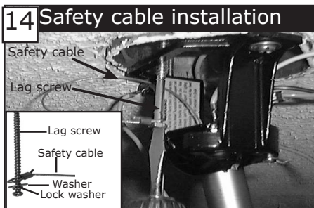
14 Safety cable installation For Canadian installation and for USA fan and light kit combinations over 35 lbs, in both flush and downrod mode the safety cable must be installed into the house structure beams using the 3" lag screws, washers, and lock washers provided. Make sure that when the safety cable is fully extended the leadwires are longer than the cable and no stress is placed on the leadwires.
