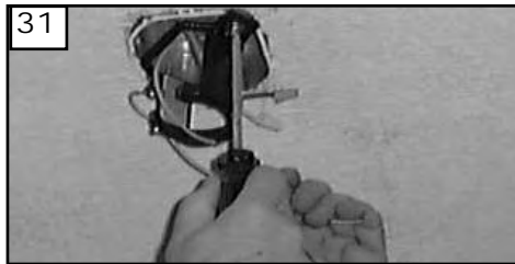
31 Use metal outlet box suitable for fan support and use only the screws provided with the outlet box (must support 35 lbs). Before attaching fan to outlet box, ensure the outlet box is securely fastened by at least two points to a structural ceiling member ( a loose box will cause the fan to wobble). Remove the two outlet box screws provided with the box, aligning the holes of the mounting bracket with the holes of the outlet box. Re-install the 2 outlet box screws securely.
