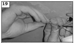
Make wire connections to power source using wire nuts provided. Make sure that no filiments are outside of the wirenut. After making the wire connections, the wires should be spread apart with the grounded conductor and the equipment-grounding conductor on one side of the outlet box and ungrounded conductor on the other side of the outlet box. The splices, after being made, should be turned upward and pushed carefully up into the outlet box.
