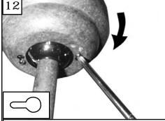
Lift canopy to ceiling aligning the key hole slots with the screws on the bottom of the mounting bracket. Rotate the canopy counter clockwise to lock in place. Tighten the screws to secure the canopy. See insert for key hole shape.
