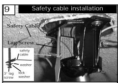
For Canadian installation and for USA fan and light kit combinations over 35 lbs, in both flush and downrod mode the safety cable must be installed into the house structure beams using the 3" lag screws, washers, and lock washers, provided. Make sure that when the safety cable is fully extended the leadwires are longer than the cable and no stress is placed on the lead-
