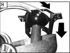
Hang assembled fan from the mounting bracket installed to ceiling in previous steps. Make sure the fan is hanging straight. Rotate fan until the tab on the Mounting bracket engages the slot on the Downrod Ball. This must be done to prevent the fan body from rotating when the blades are in motion.
