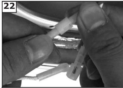
22 Connect white wire from fan to white wire from light fixture. Then plug blue wire from fan to black wire from light fixture by pushing together the connectors.
