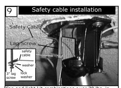
Fan and light kit combinations over 70 lbs, in both flush and downrod mode the safet y cable must be installed into the house structure beams using the 3" lag screws, washers, and lock washers, provided. Make sure that when the safety cable is fully extended the lead wires are longer than the cable and no stress is placed on the lead wires.
