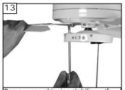
Remove any shipping stabilizers if present. Attach blade assembly to motor using the motor screws and washers provided. Tighten screws securely.
