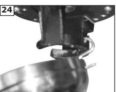
Hang fan from mounting bracket by the hands free "S" hook in hardware pack into a closed hole on the edge of the canopy and over bracket.. Note: For Canadian mounting refer to Step #10.
