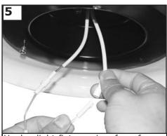
Unplug light fixture wires from fan wires.
