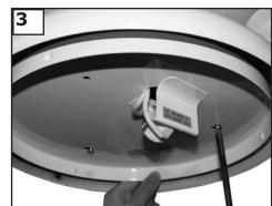
Remove light fixture by loosing 2 screws with key slots and remove 1 screw without key slot. Save screw.
