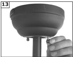
Next lift the canopy disk and install knurled nuts as shown. Tighten the knurled nuts securely. The canopy should adjust for any irregularity in the ceiling or Outlet box.
