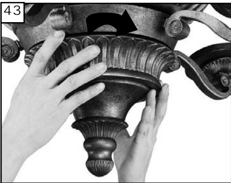
43 Raise decorative cover and twist clockwise until tight.
