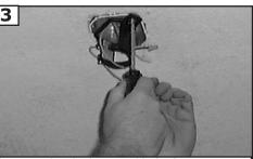
Use metal outlet box suitable for fan support and use only the screws provided with the outlet box (must support 35 lbs). Before attaching fan to outlet box, ensure the outlet box is securely fastened by at least two points to a structural ceiling member ( a loose box will cause the fan to wobble). **Use only the screws provided with the outlet box.**
