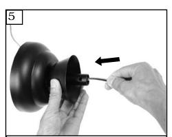
Thread wires and safety cable through downrod with canopy and yoke cover assembled.
