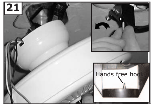
21 Remove the all thread studs from the lower part of the mounting bracket. Hang fan from mounting bracket by the hands free hook into a closed hole on the edge of the Canopy. Note: For Canadian mounting refer to Step #8.
