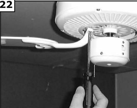
Install blades to motor using the 10 motor screws provided. Tighten screws securely.
