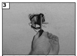
Install the Mountiing Bracket to the Outlet box. **Use only the screws provided with the outlet box.**
