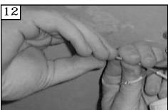
Make wire connections to power source using wire provided. Make sure that no filiments are outside of the wirenut. After making the wire connections, the wires should be spread apart with the grounded conductor and the equipment-grounding conductor on one side of the outlet box and ungrounded conductor on the other side of the outlet box
