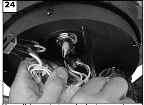
24 Install by twisting clockwise, replace screw removed from motor plate. Tighten all 3 screws securely.
