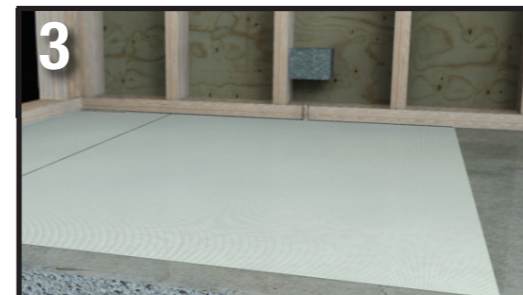
3 FloorWarm is wired to a junction box.
