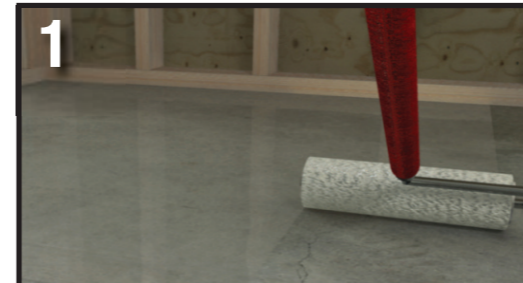
1 Roll on FloorWarm #6000 Primer, allow 20-30 minutes to dry.
