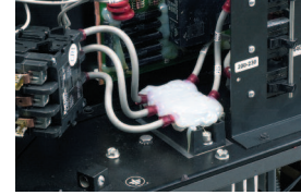
Coated Electrical Connections
