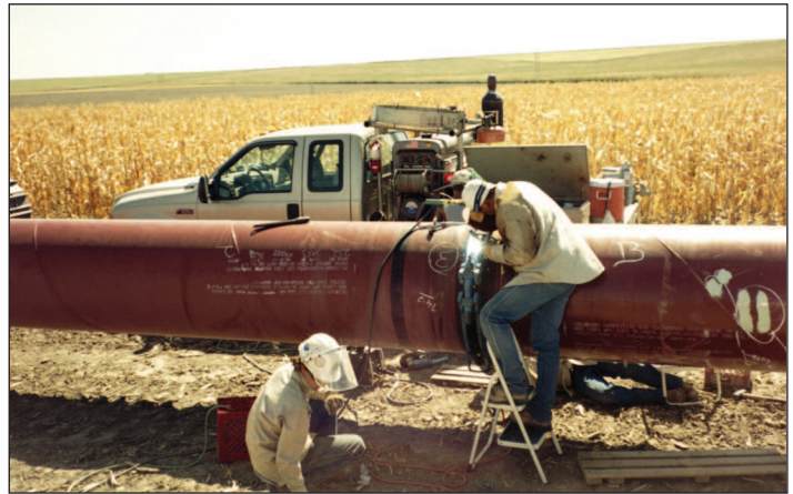
Cross-country pipe welding with Classic® 300D.
