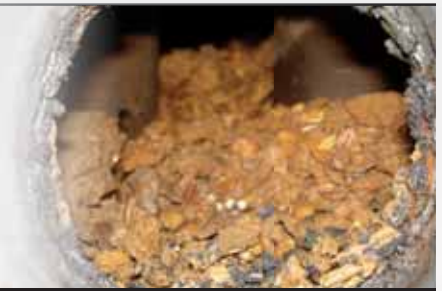
“In-tank” flue tubes and heat exchangers suffer from lime scale buildup beginning from the first hours of operation.
