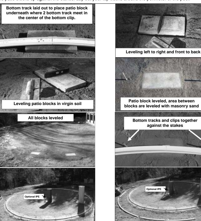
All blocks are leveled, bottom track and clips put back together against the stakes in the ground. Place top track around the pool perimeter, place wall, Opt. IPE roll, rakes, shovels, tamper, and 4'x4' wall boards to the inside of the pool. Have all tools, hardware and insulation ready for installation.
