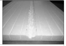
Last piece needs to be cut, make a straight line and cut with a utility knife and slide in. Be sure it's a tight fit.
