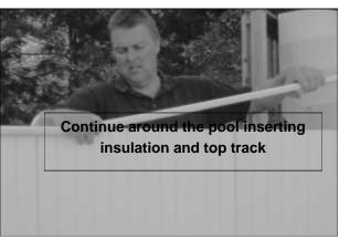
After bolting the wall you will prepare the last 2 pieces of insulation, one will be cut to size and one will be notched for the bolting pattern
