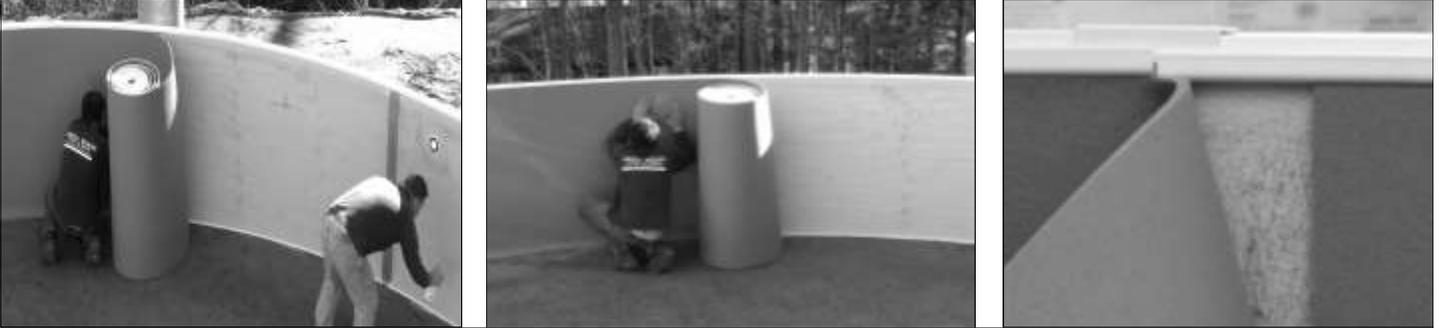
Cut through both layers at the same time, remove inside piece and place 3 layers of duct tape on the seam
