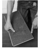
This space must also be provided at all columns, heating pipes, steel doorframes, etc. The planks are laid with the tongue side facing the wall to be able to work with the tongue/groove system.
