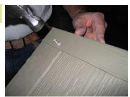
Install aluminum corners on top for the ridge and fasten with white trim nails as shown.
