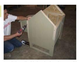
Attach the wall with the wheels and secure with 1 1/4" screws as shown.
