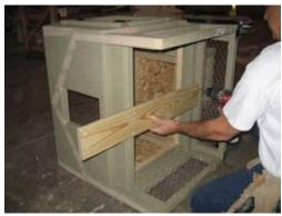
Install the chicken ramp. Secure with 2 1/2" screws. Two in the back and two in the front.
