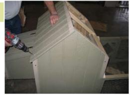
Install roof, Make sure roof overhangs 1" on sides, and secure with 1 1/4" screw.
