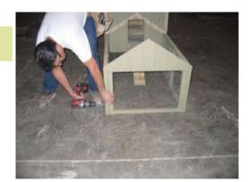
Secure with 2 1/2" screws as shown.
