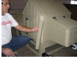
Install aluminum corners on the outside as shown and secure with white trim nails.
