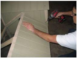
Next install the roof on the lower section. Secure with  $1 \frac{1}{4}$  screws.
