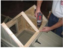
Next locate the rafters and secure with 1 1/4" screws.
