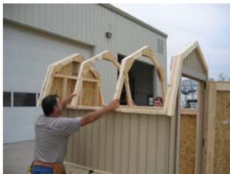
Now install trusses.
