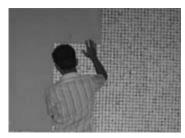
When done, use grout to fill up the spacing gaps (you can use sealant if you choose spacing gaps of 1-2 mm). And remove unnecessary overflows by damped clothes.
